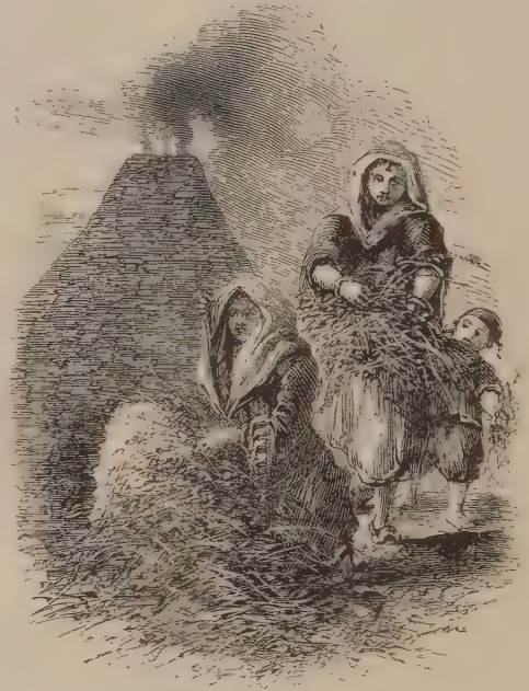
HEATING OVENS WITH DRY GRASS.
